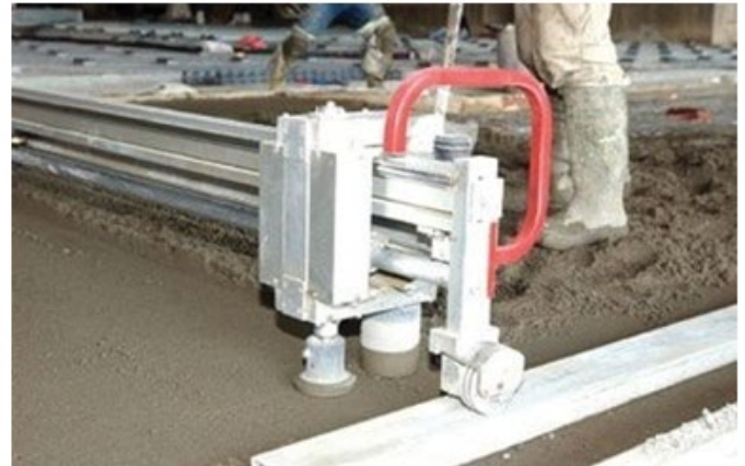
Figure 1. Automatic concrete screeding machine.
