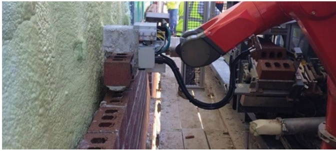
Figure 5. Automated brick masonry laying robot.
