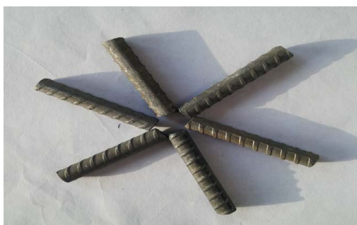
Figure 2: Steel embedded in concrete with 0.5% of hexamine after 90 days exposure.
