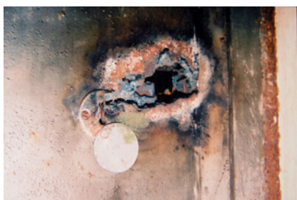
Figure 4: Strong room door with the steering wheel.
