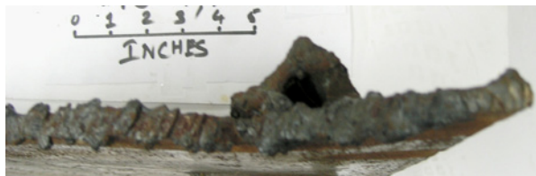
Figure 13: The gas cut tool marks on the piece of the strong room door.
