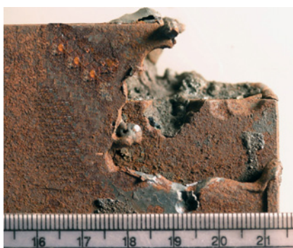
Figure 6: Part of the lock damaged.
